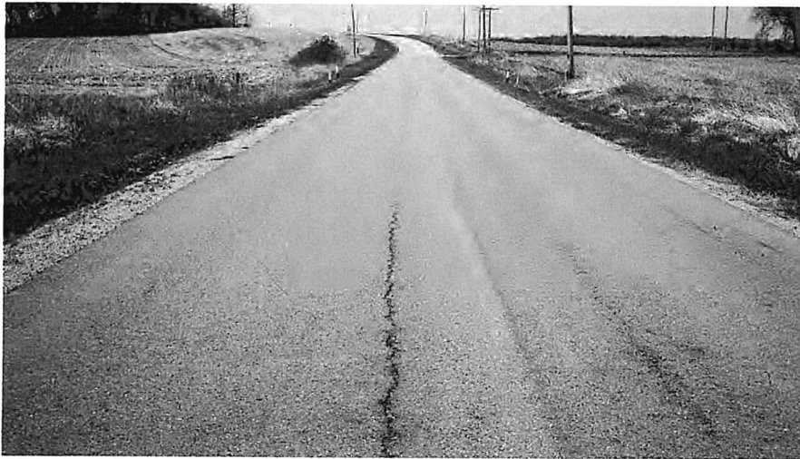
▼ Slight rutting; patch in good condition.
