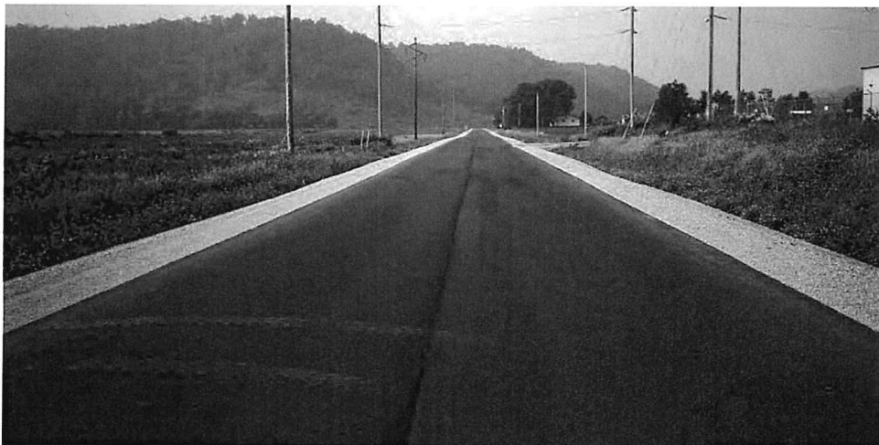
▶ RATING 9 Recent overlay, rural.
