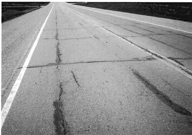
Load-related cracks in wheel path. ▼
