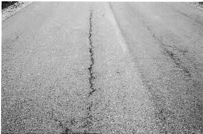
Multiple open, longitudinal cracks that are raveling. ▼
