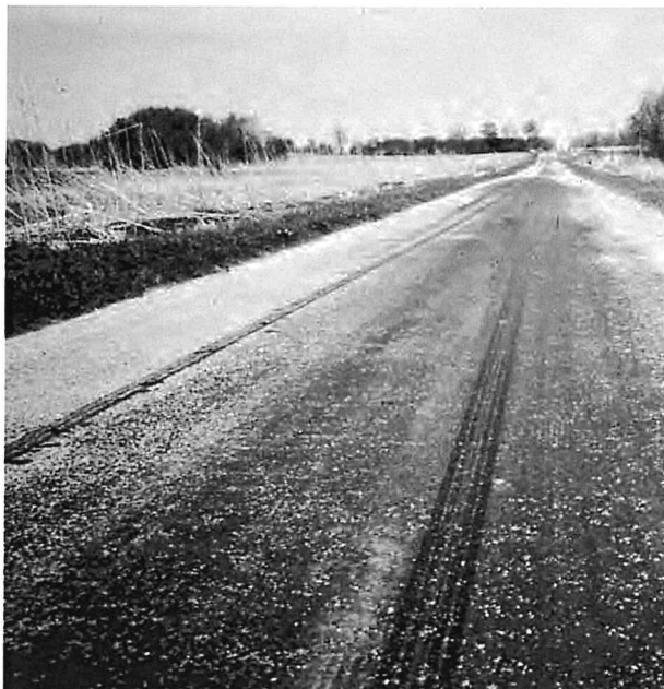
▼ Severe flushing.
