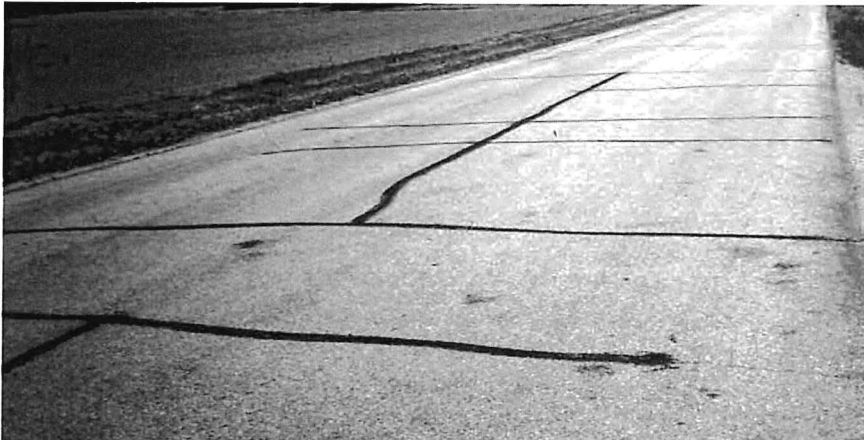
▼ Open crack, 1/2" wide; adjoining pavement sound.
