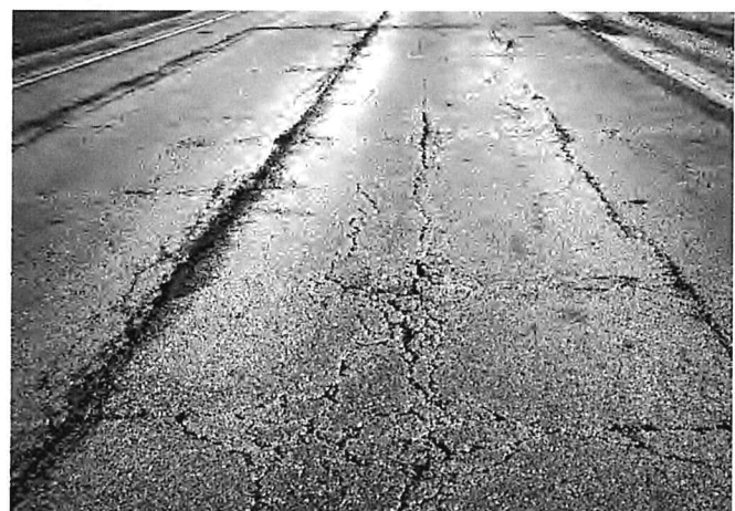
Multiple open, longitudinal cracks that are raveling. ▼
