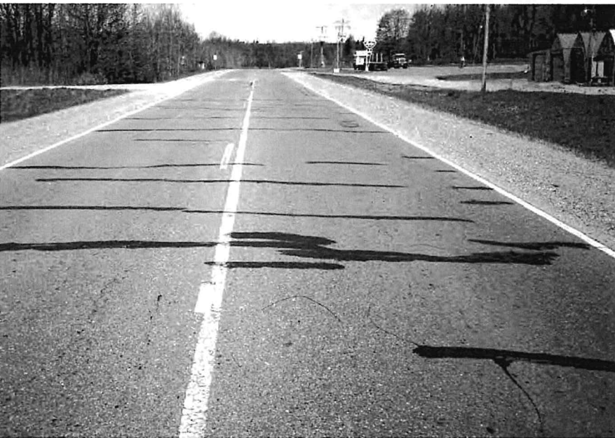
◀ Sealed cracks, a few feet apart.
