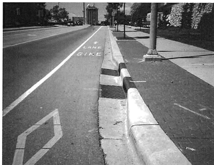
Urban drainage. RATING: Excellent
