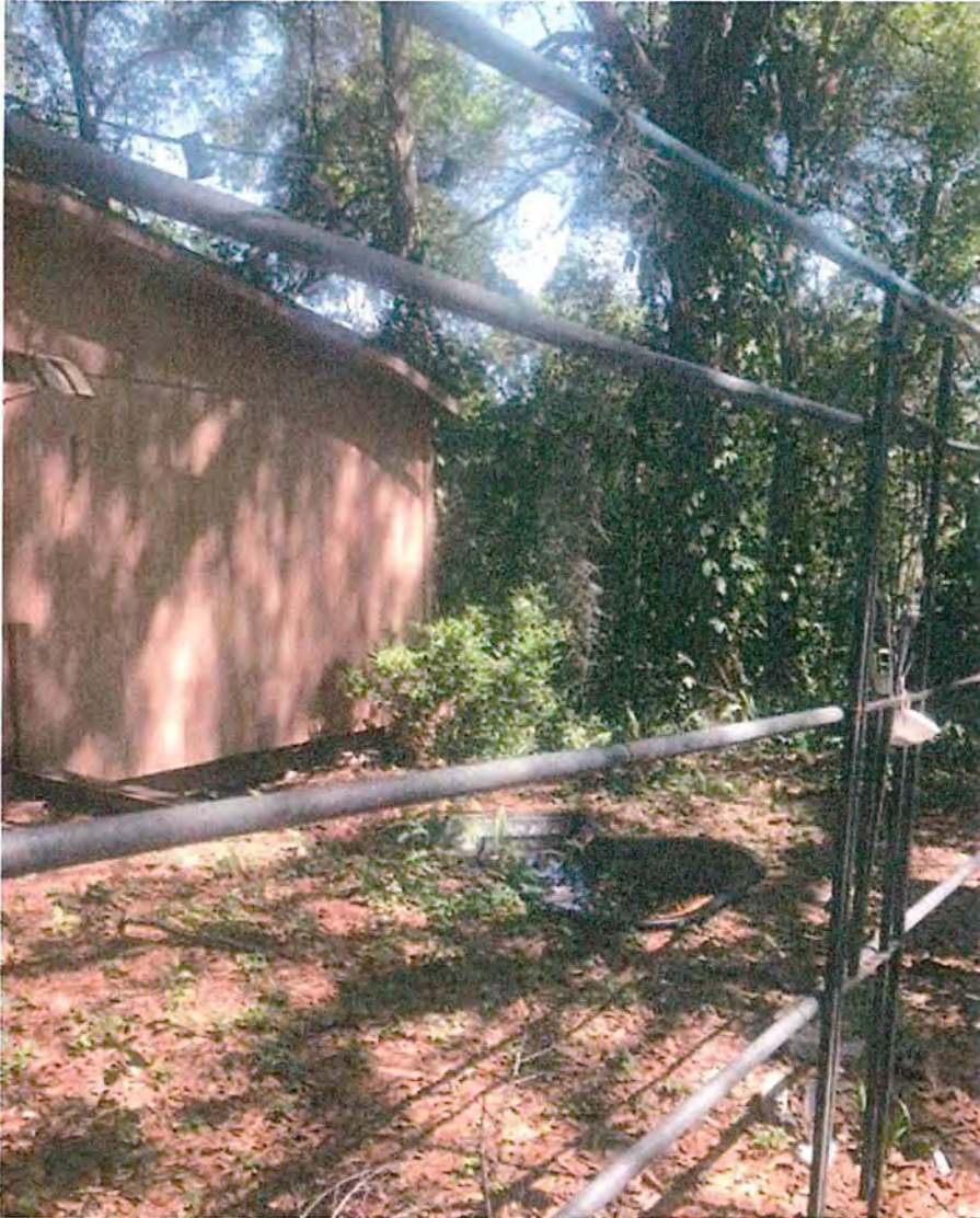
FRONT & EAST SIDE VIEW OF PROPERTY: MIXTURE OF FENCING MATERIAL
