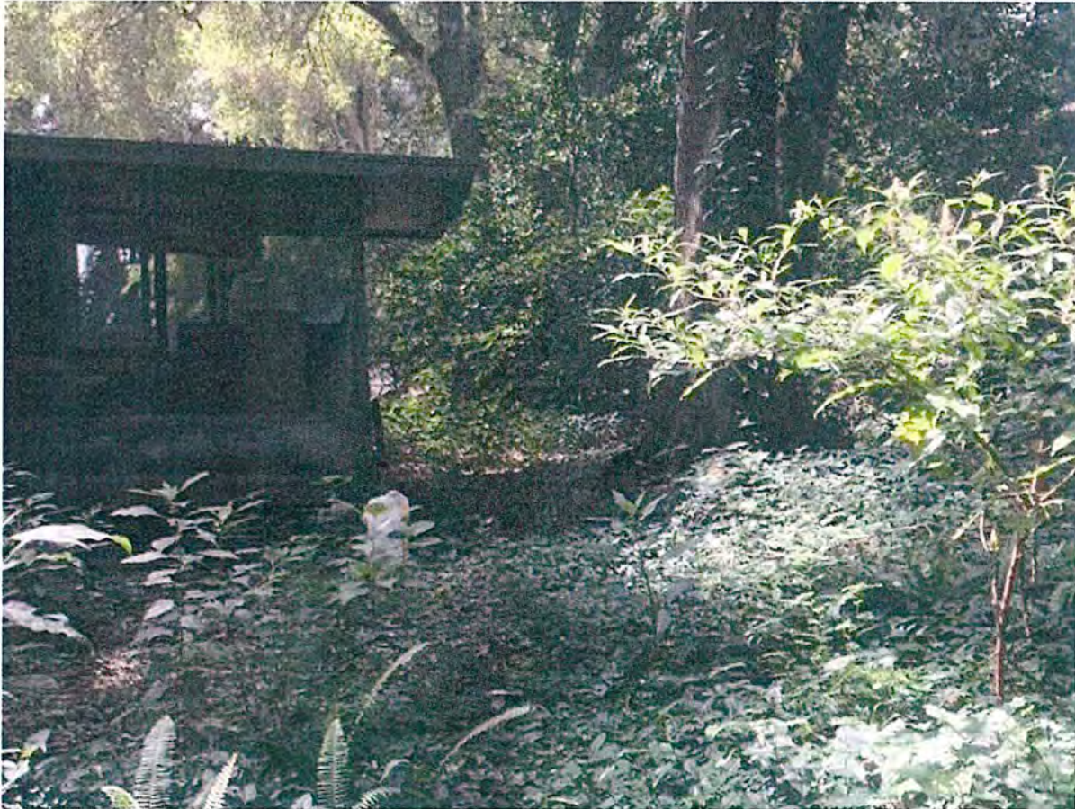
SOUTH SIDE VIEW OF PROPERTY: VEGETATION OVERGROWTH
