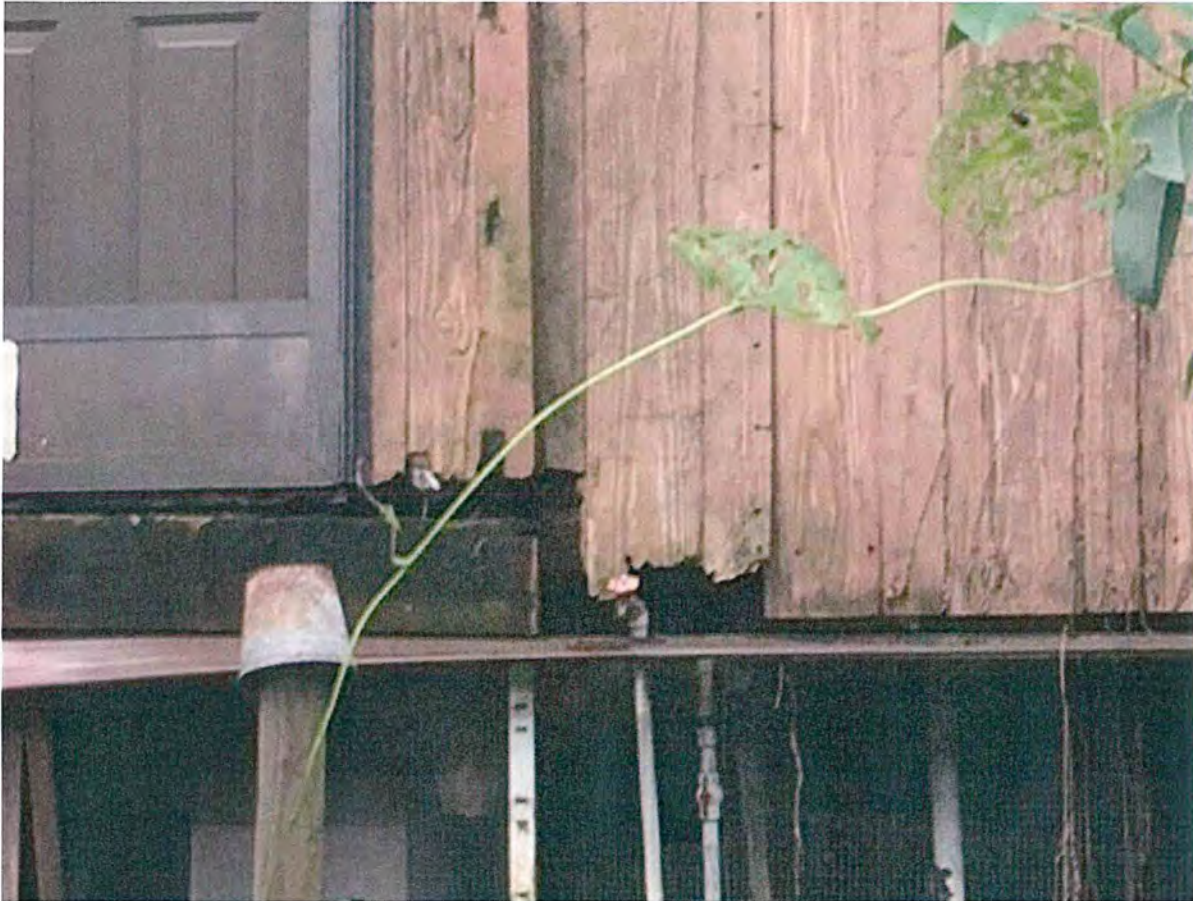
RIGHT & NORTH SIDE VIEW OF MOBILE HOME: EXIT DOOR CLOSE UP
