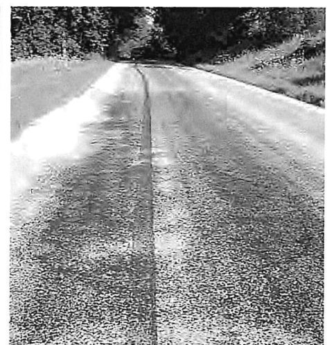
▼ Moderate flushing.
