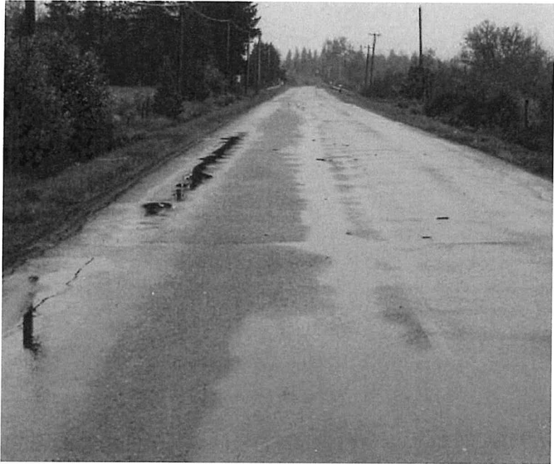
◀ Even slight rutting is evident after a rain.
