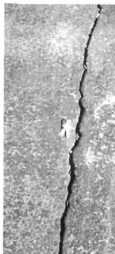
▼ Open crack, 1/2" wide; adjoining pavement sound.
