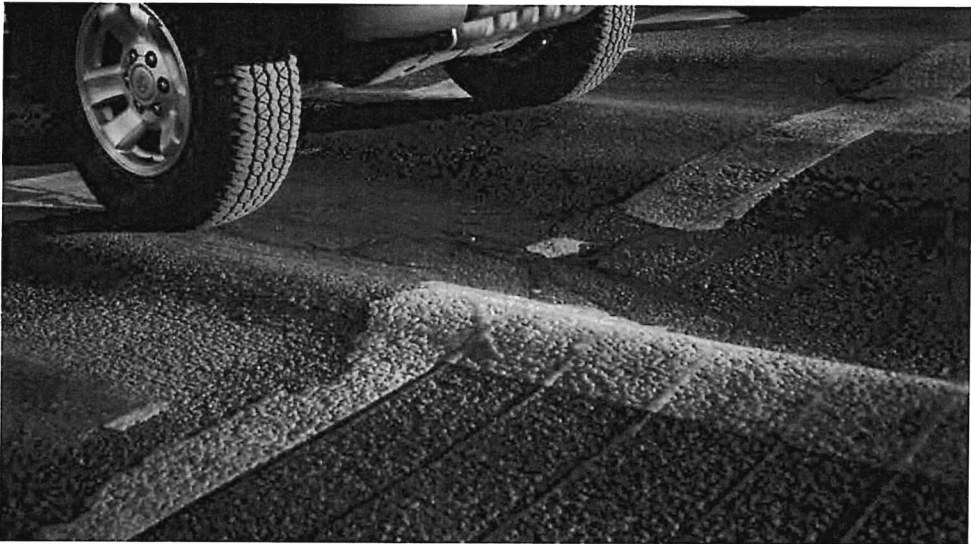
◀ Even slight rutting is evident after a rain.
