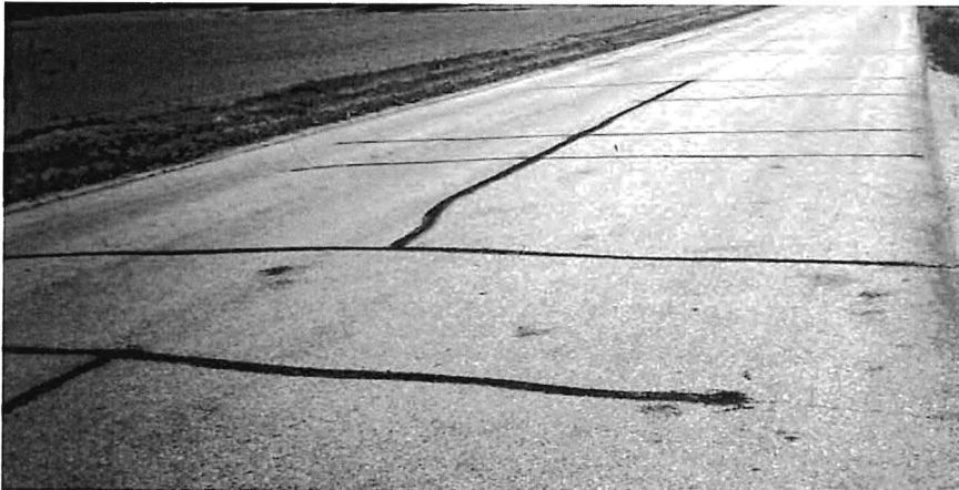
▼ Open crack, 1/2" wide; adjoining pavement sound.
