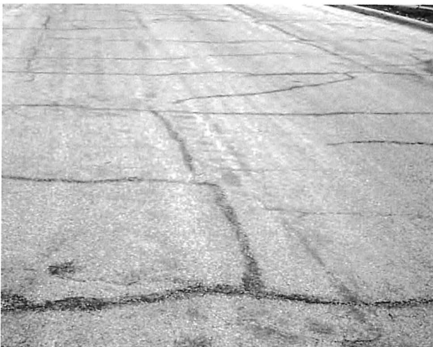
▼ Large blocks, early signs of raveling and block cracking.
