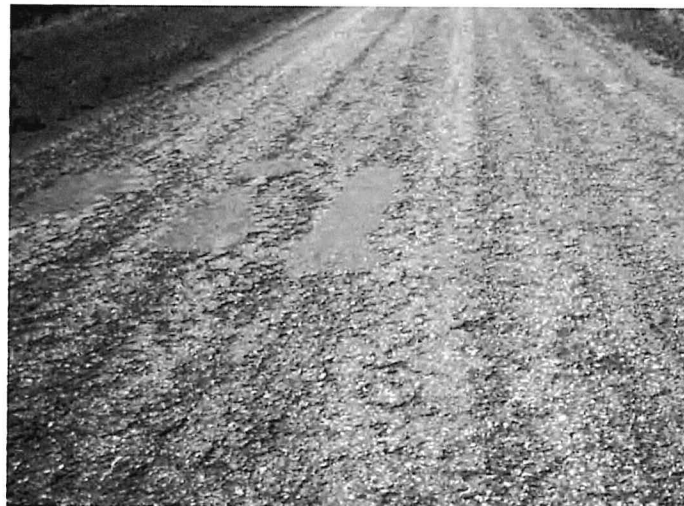
Polished, worn aggregate needs repair. ▼
