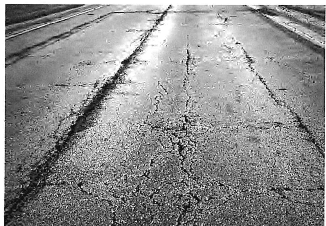
Multiple open, longitudinal cracks that are raveling. ▼
