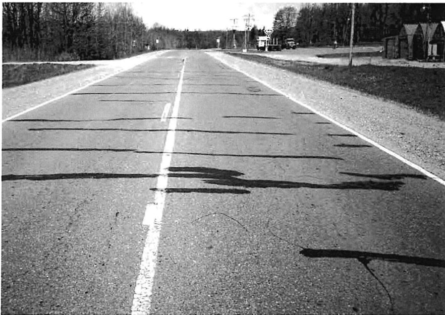
◀ Sealed cracks, a few feet apart.
