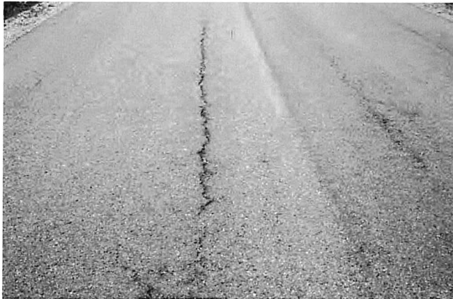
Multiple open, longitudinal cracks that are raveling. ▼
