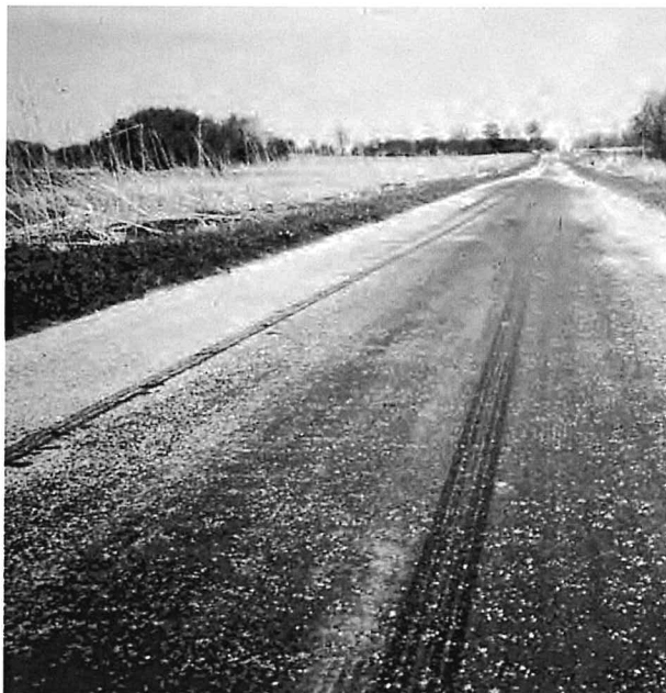
▼ Severe flushing.
