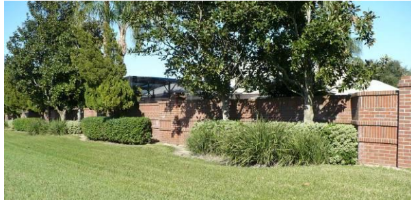
Use of durable materials, jogs in the wall and landscaping to provide interest
