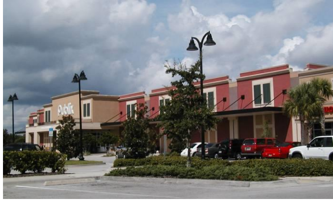
Use of false windows and shutters to provide architectural interest
