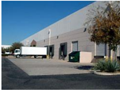
Undesirable loading dock facing street with unscreened refuse container
