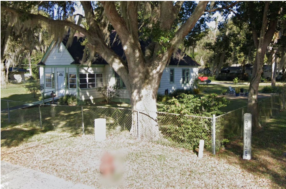
Figure 4. Fountain Street, street marker and structure (image courtesy of google street view).
