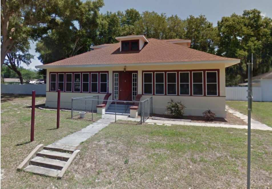
Figure 3. South Dixie Avenue structure (image courtesy of Google street view).
